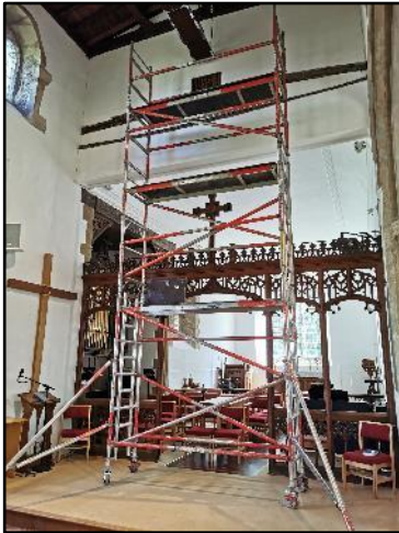
Accessing the heating system
